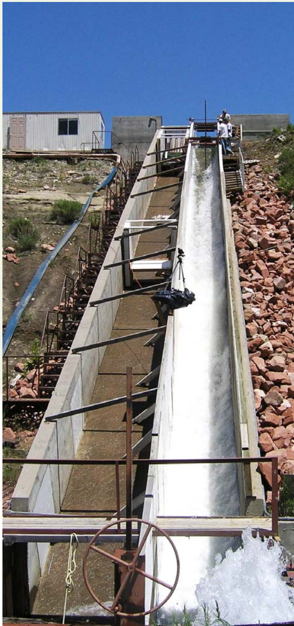
10-ft outdoor flume configured to a 4-ft channel width conveying 86 cfs with a corresponding overtopping depth of 3 ft.
